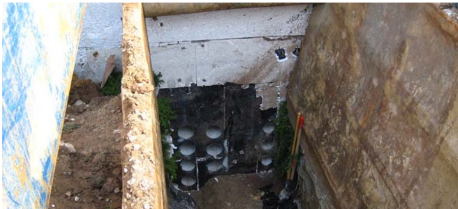
Looking east into the tunnel trench at utility connections to the adjacent Cancer Research Building I
