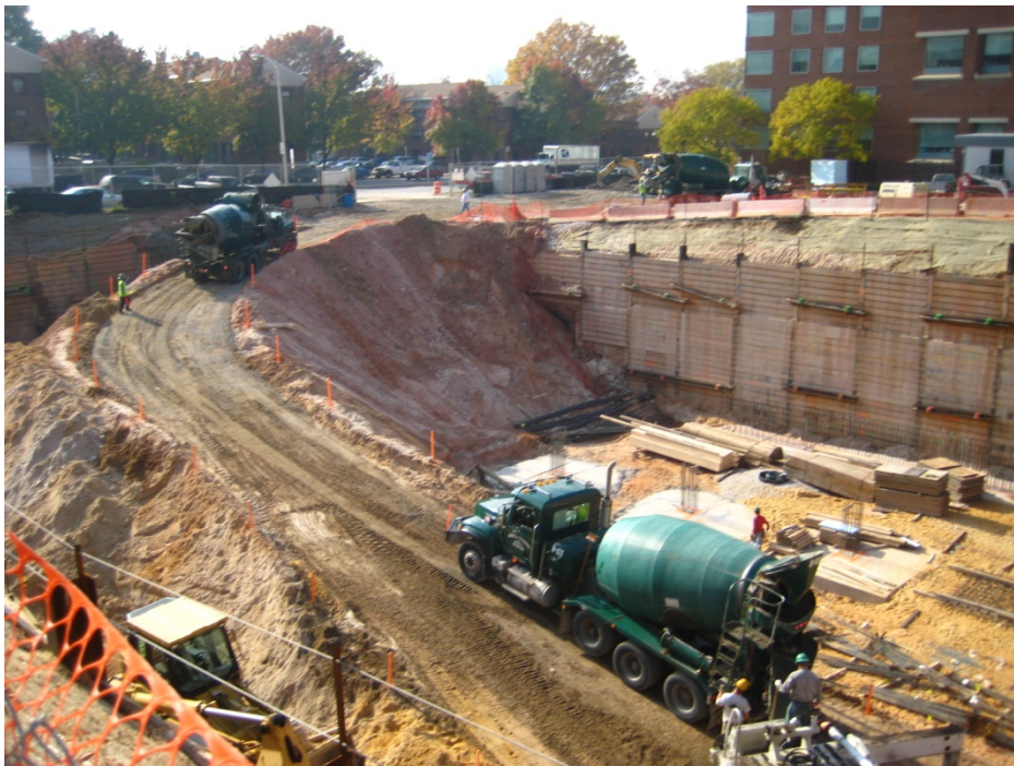
Temporary excavation ramp to be removed.
