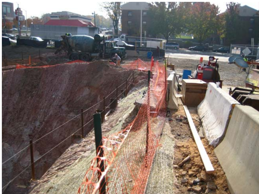
Looking south from site
