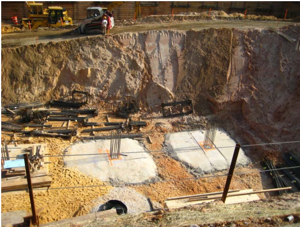
Completed column footings
